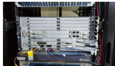
Gambar 2. SDH Huawei
