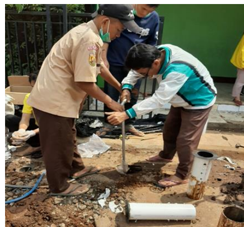
Figure 4. make biopore infiltration holes
