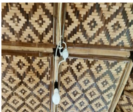
Fig. 9 Unstandard Installation Repair
