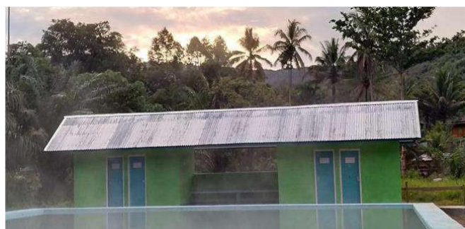
Fig 17. Toilet and changing room
