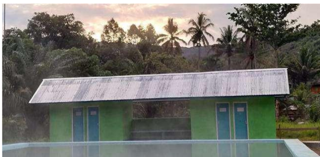
Fig 17. Toilet and changing room
