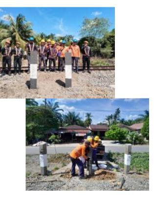
The installation of concrete pads by PT KAI is carried out in a measured manner, considering the appropriate distance and height to prevent access for four-wheeled vehicles, while still allowing pedestrians and two-wheeled vehicles to pass. PT KAI must continue to conduct regular evaluations to ensure the optimal function of the concrete pads without causing new problems for the surrounding community.
