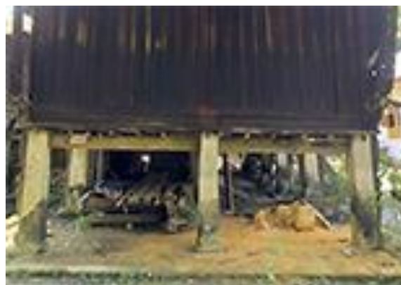
Figure 7. Girders construction of the Bawi Malay Tribe Lontiok house
