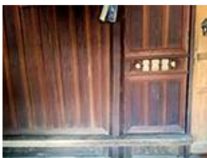
Figure 11. The interior wall construction of the Bawi Malay tribe's Lontiok house
