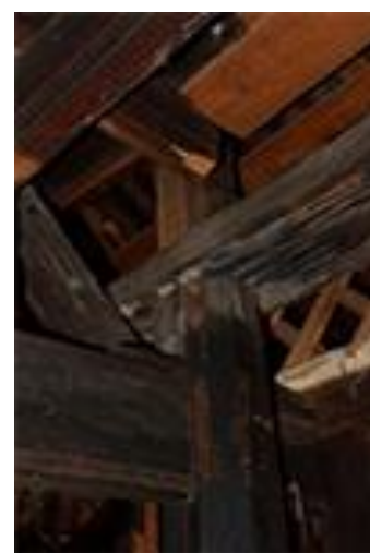
Figure 9. The Lontiok house connection system of the Bawi Malay people Source: Personal documentation, 2022
