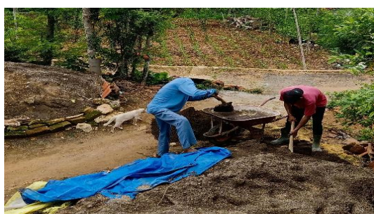
Image 4. House Renovation (Casting Process Using Sand and Cement)
